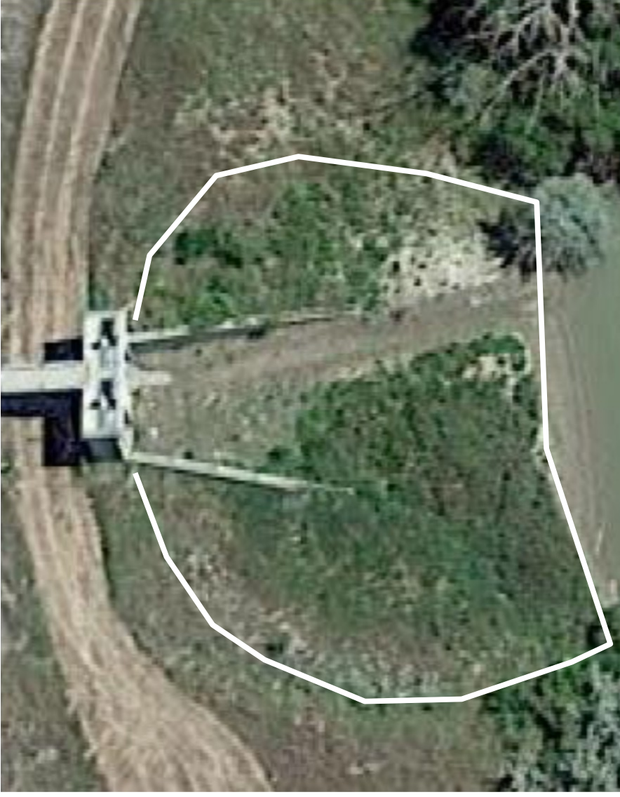
Station 258 Stilling Basin
